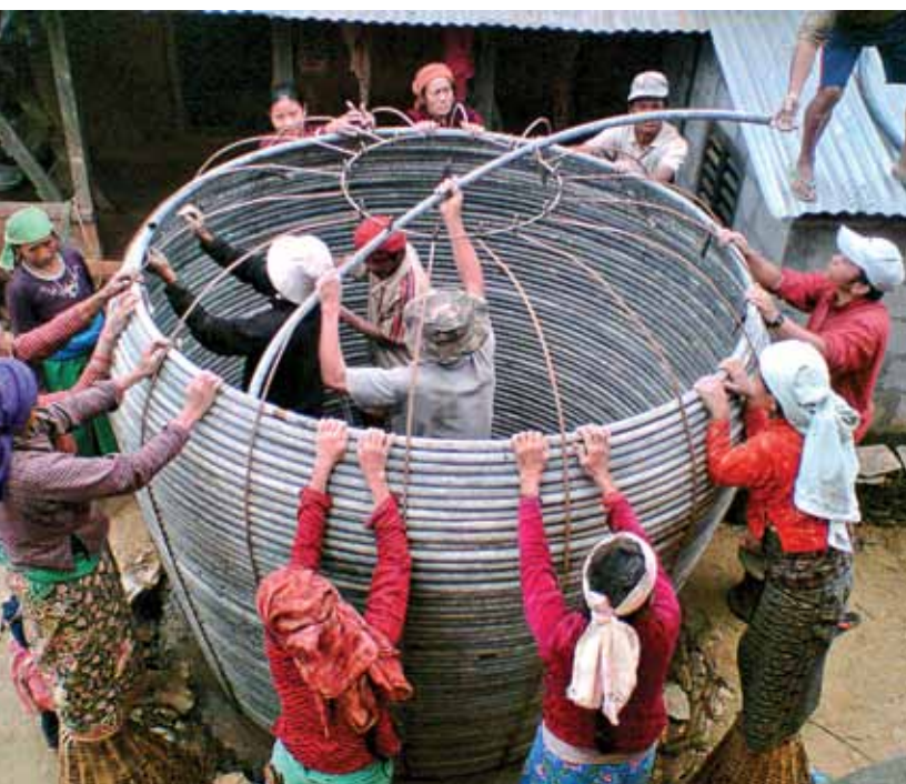
Service providers at work: construction of Rainwater Jar
