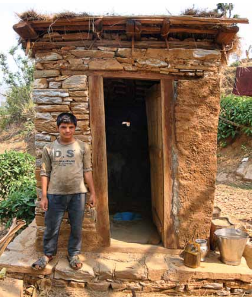
A household toilet in the rural village
